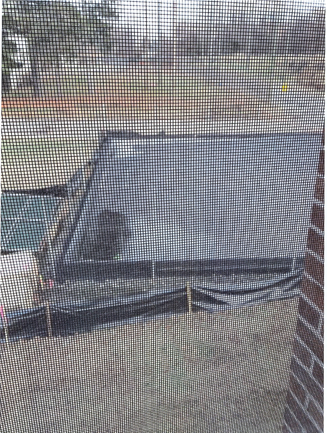
Waste Storage Area, not yet completed, outside my North window 20 feet from my house
