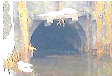
Photo 3: North View of Open Gate
