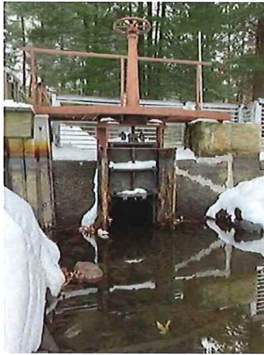
Photo 15: North View of Outlet Gate Structure
