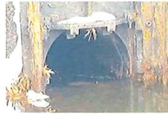
Photo 16: North View of Open Gate
