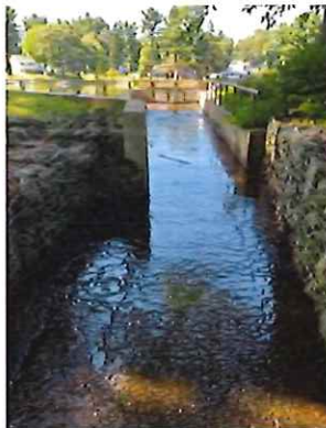
Photo 1: South View of Spillway Outlet
