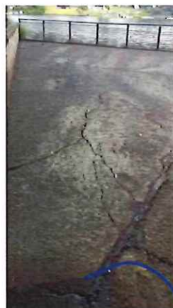
Photo 2: South View of Spillway
