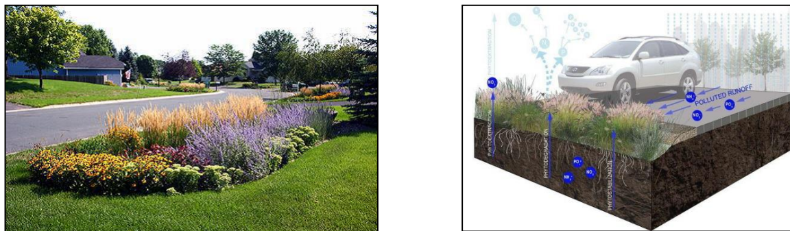
Figure 3-A. Photo of a Rain Garden and LID Parking Lot Storm Drainage
